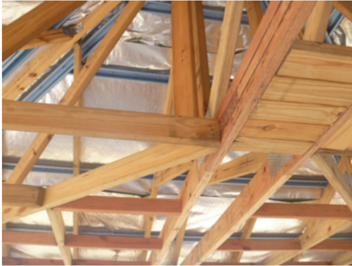
Detail E2 - Jack Truss to Hip Truss (maximum jack station 2400mm)
