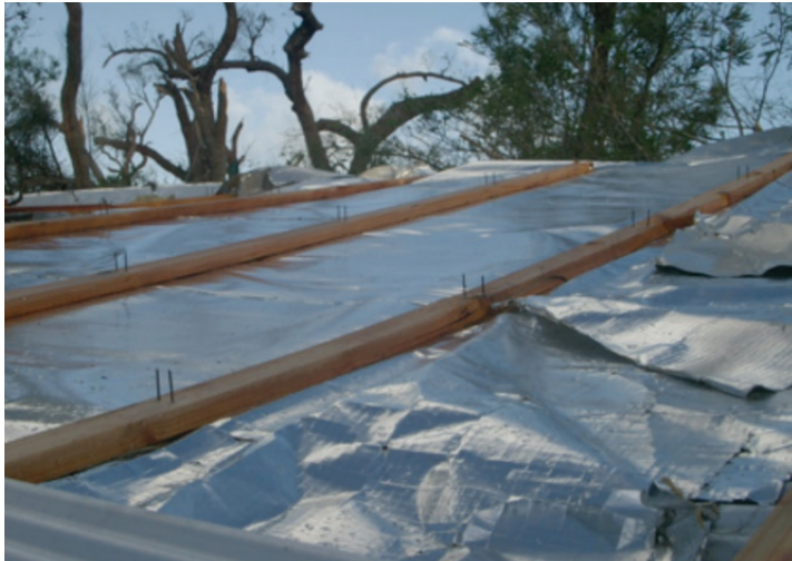
Photograph 5 – Roof sheeting and battens have failed due to nailed batten fixing where screws should have been used
