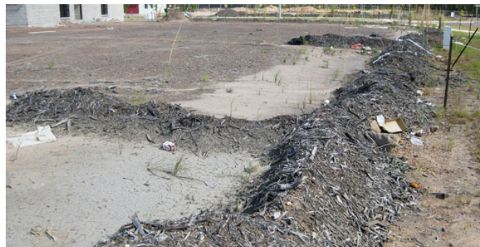
Mulch berm with upslope 'return' being used on small, flat house lots. (Source: Catchments and Creeks Pty Ltd)
