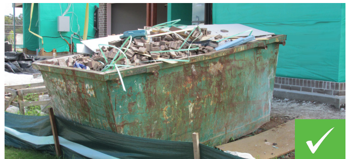
Keep all rubbish in skip bins or mesh cages. (Source: Healthy Land and Water)
